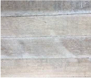
Small cracks due to temperature & humidity variations
