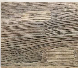
Blocking to replace holes left by hardware.
